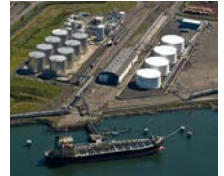
Bulk Liquids being exported from the Port of Grays Harbor
